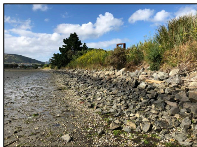
Rip rap wall in western Onepoto arm
