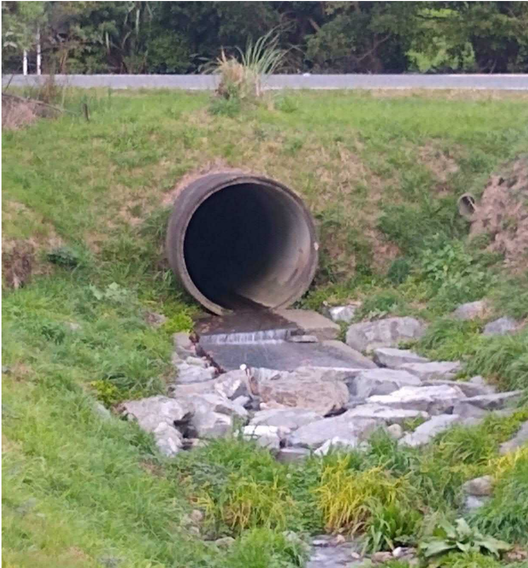
Figure 13. Dry weather discharge from a stormwater culvert draining to Te Awa Kairangi (the Hutt River), likely from groundwater infiltration or leakage from the potable network.
