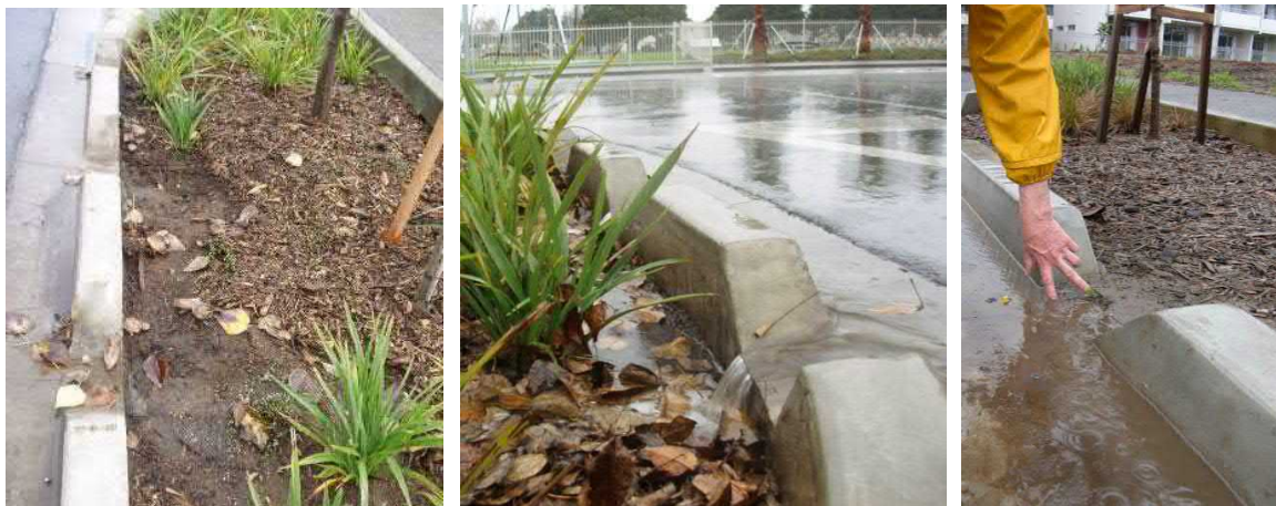
Scouring at raingarden inlets displaced mulch and soil (left). Stormwater inflow showing concentration of water to one side of the cut, but no scouring or leaf litter displacement (centre) and stormwater prevented from entering the raingarden due to overfilling with media/mulch (right). All photos in June/July 2008.
