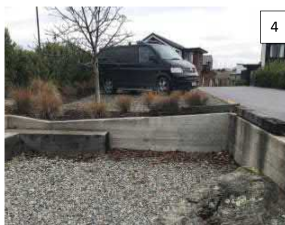
Photo 1: Stage 1 Rain gardens shortly after construction, before house construction showing raised edges.
