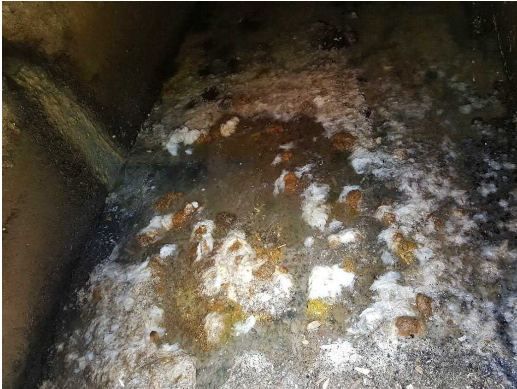
Figure 2. While shocking, this is the reality of an illegal cross connection in Te Aro (Wellington City) from a private residence, where their waste was being routed to a stormwater main. The next rainfall event would transport this to Wellington Harbour. Image courtesy of Steve Hutchinson (Wellington Water).
