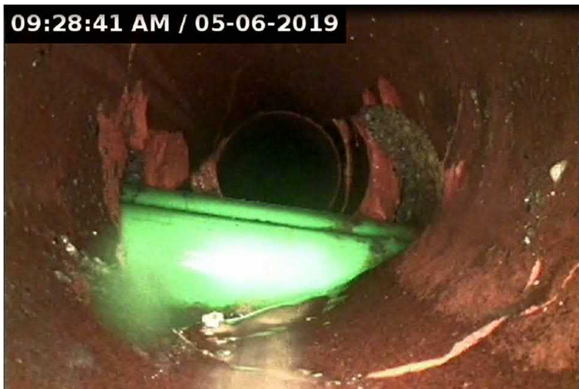
Figure 11. Strikethrough CCTV image within a wastewater pipe. Image courtesy of Steve Hutchinson, Wellington Water
