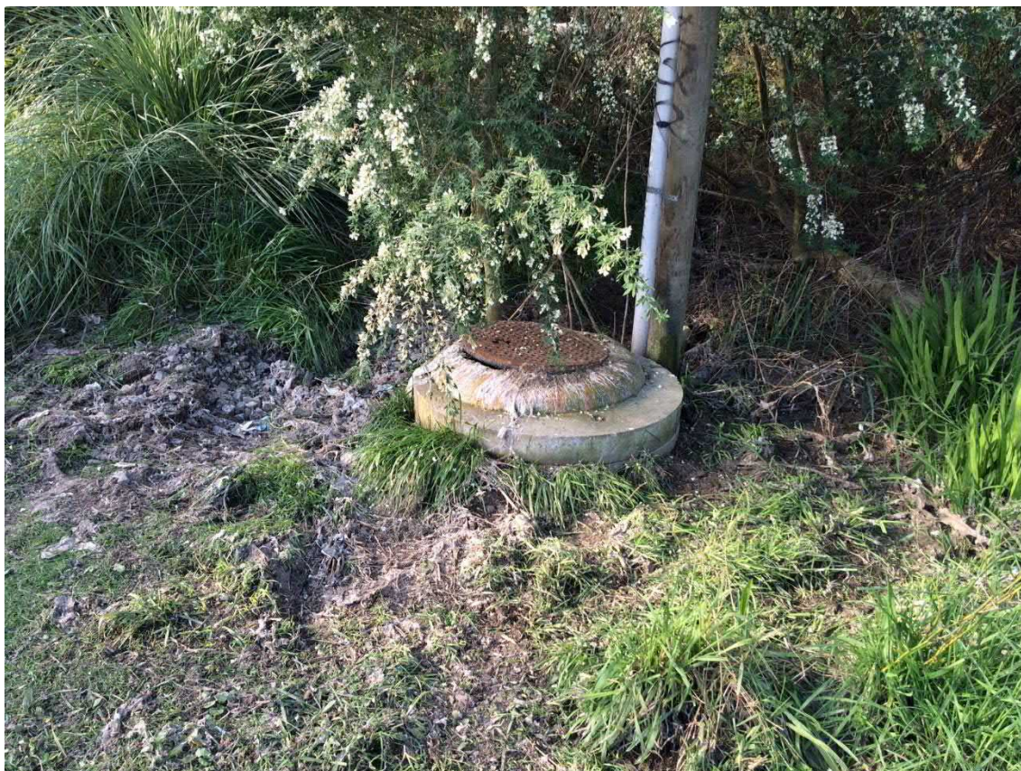
Figure 9. Un-constructed raw wastewater overflow discharging to the environment. Image courtesy of Steve Hutchinson, Wellington Water.
