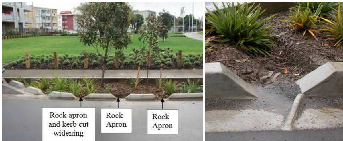
Solutions identified to scouring issues, June 2008. At this stage most groundcover plants and trees were about 18 months old, but the tree on the right is new (left). Overfilled rain garden with concrete gutter 'wing' to improve runoff entry (2008) (right).
