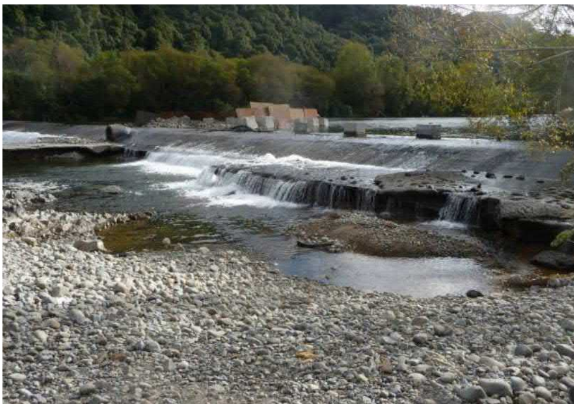
Figure 8. Silverstream weir and constructed overflow. Image courtesy of Shearer (2017).
