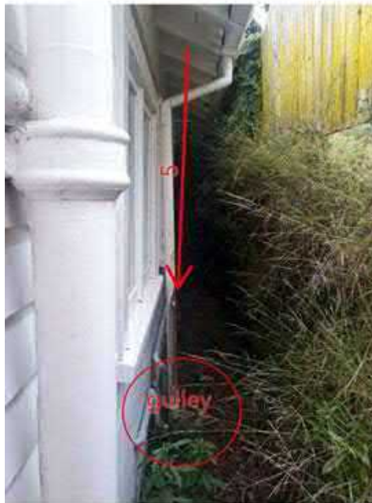
Figure 1. Inflow from a residential property where the down pipe has been routed to a gully trap (connecting to the wastewater network). Image courtesy of Steve Hutchinson, Wellington Water.
