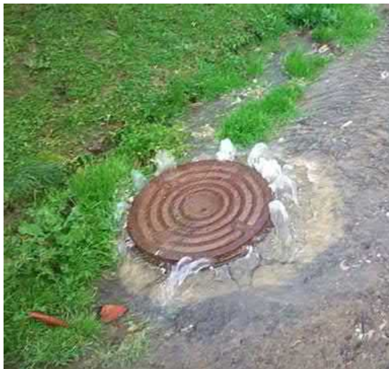
Figure 3. Un-constructed overflow occurring from a manhole lid. Image courtesy of Steve Hutchinson, Wellington Water.
