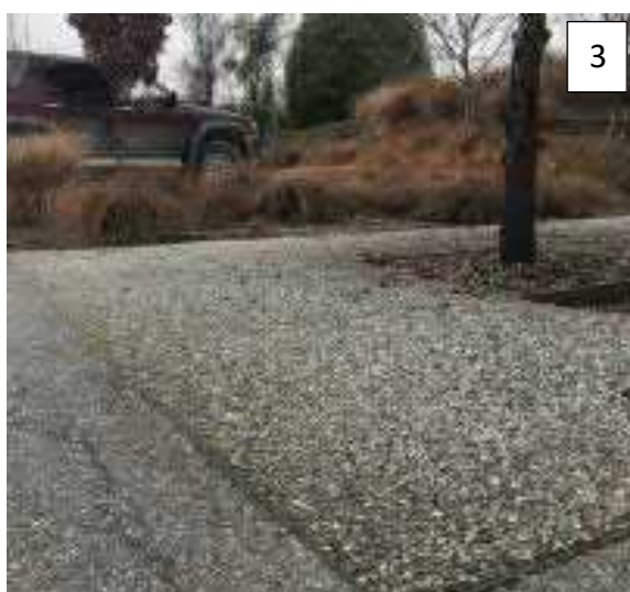
Photo 1: Stage 1 Rain gardens shortly after construction, before house construction showing raised edges.
