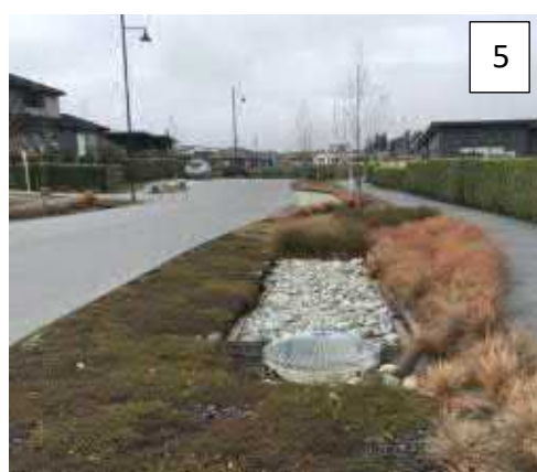
Photo 5: Raingarden with unplanted stone mulch and exposed overflow dome.
