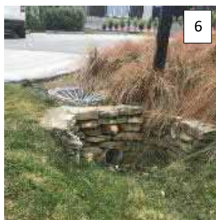
Photo 5: Raingarden with unplanted stone mulch and exposed overflow dome.
