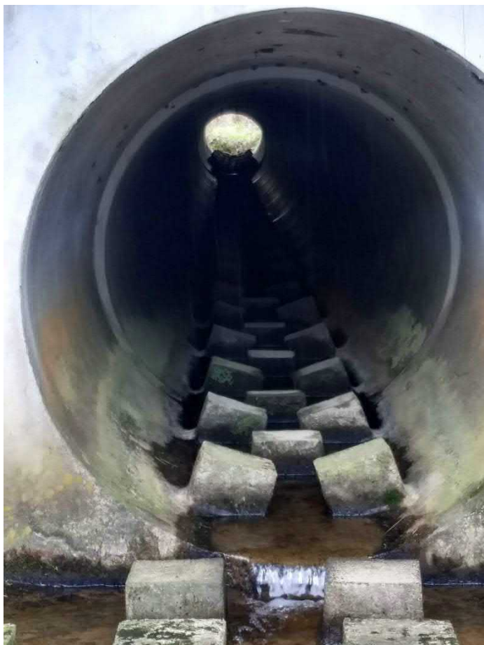
Figure 14. Culvert providing fish passage. Stormwater structures can also act as ecological barriers when fish passage hasn't been considered, or erosion and hydrological modification has happened over time.
