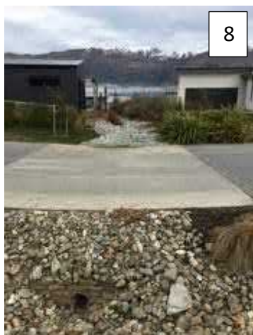
Photo 8: Fords for overland flow paths reduce need for pipes and are traffic calming features.
