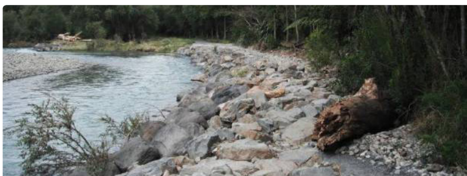
Frequent flooding over spring/summer turned the Kebbles Bend Trail beside the Waikanae River into a boulder field.
