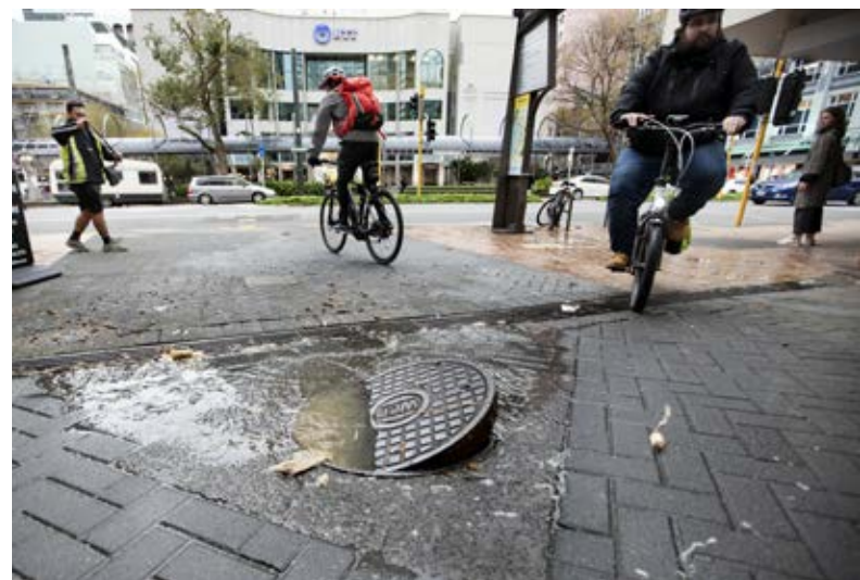
Sewage leak spill, Woodward Street, Wellington – Photo: Stuff Limited
