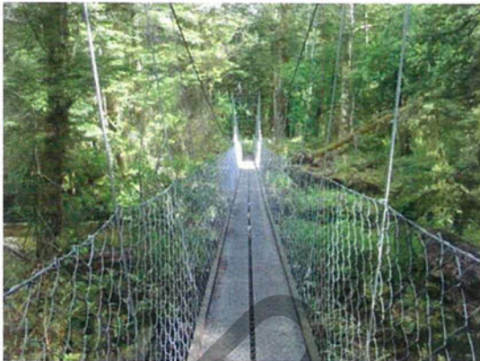
36 Potential for swing bridge across Whakatikei River below proposed dam to provide alternative loop track and views up river
