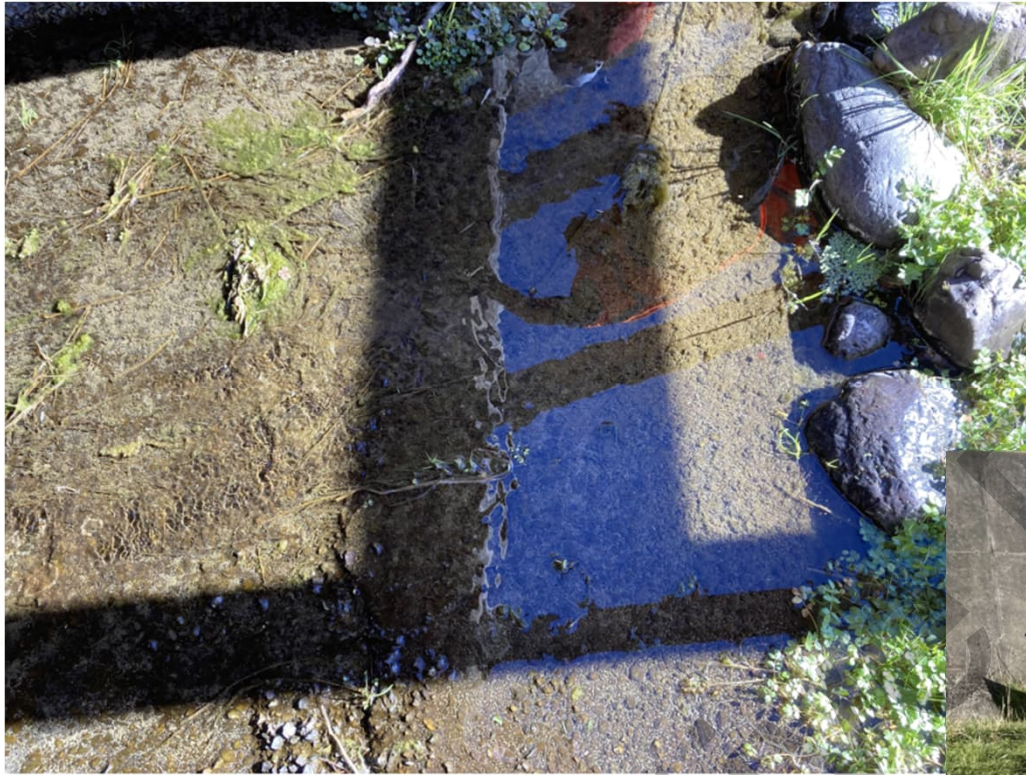
Sediment at base of left culvert (~7cm thick near downstream end)
