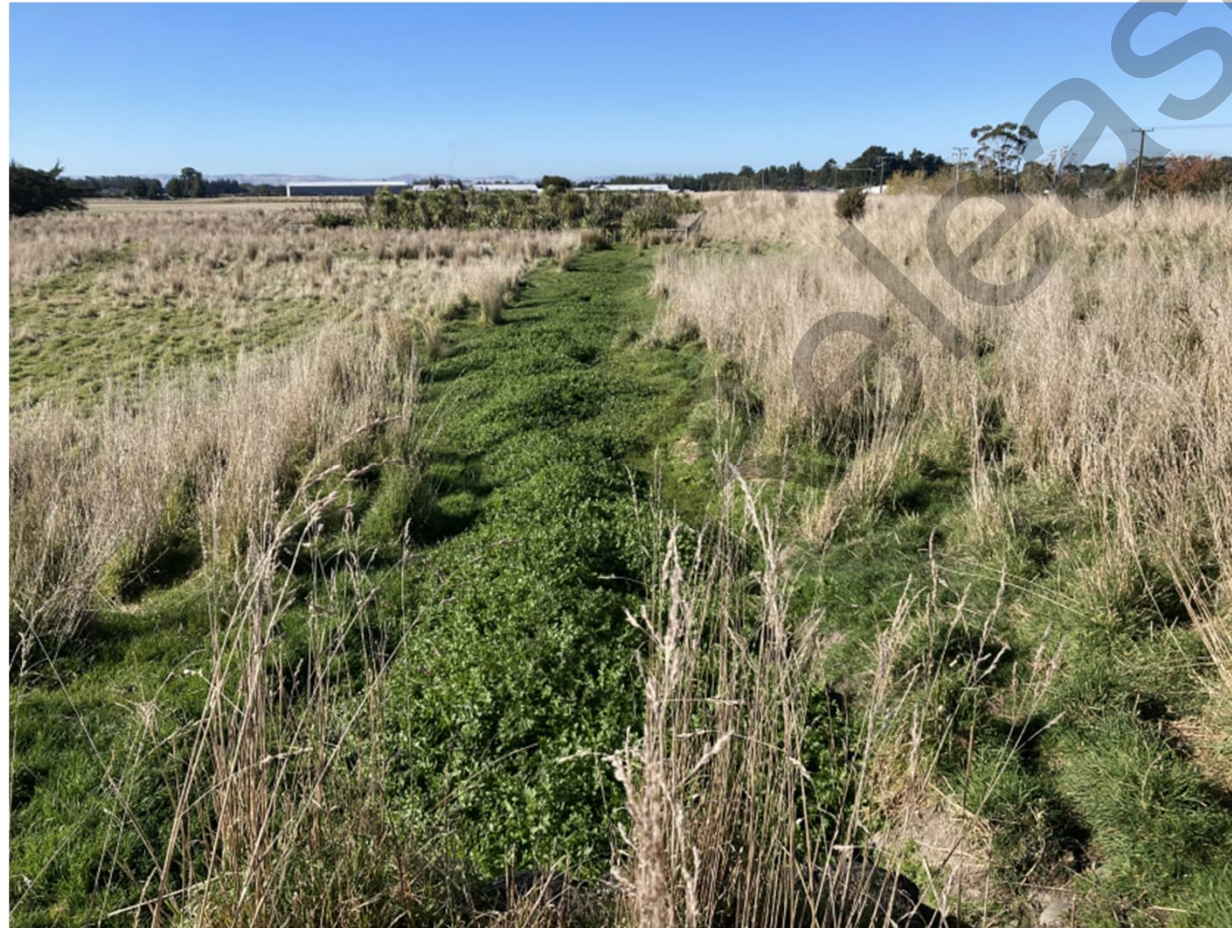
Drain along upstream toe of right embankment
