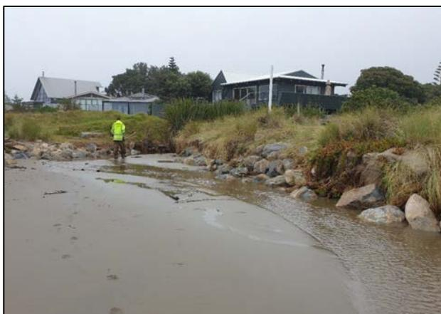
Artificial boulder field installed at Riversdale Central to minimise erosion of the dune (A12; Appendix 1; photo: April 2022)
