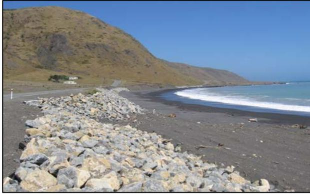
Rock armouring to prevent erosion near roading infrastructure (photo: December 2006; Wriggle Coastal Management)
