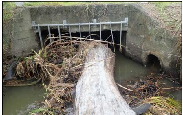
Significant build up of woody debris at the road culvert, pooled water has poor water clarity
