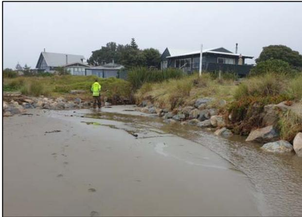
Entrance of Riversdale Centre Stream (top) and looking upstream (bottom) artificial boulders on both banks to limit erosion
