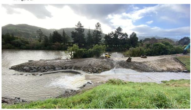
Figure 1: Stokes Valley Stream mouth showing the stream diversion and reinstated training bank
