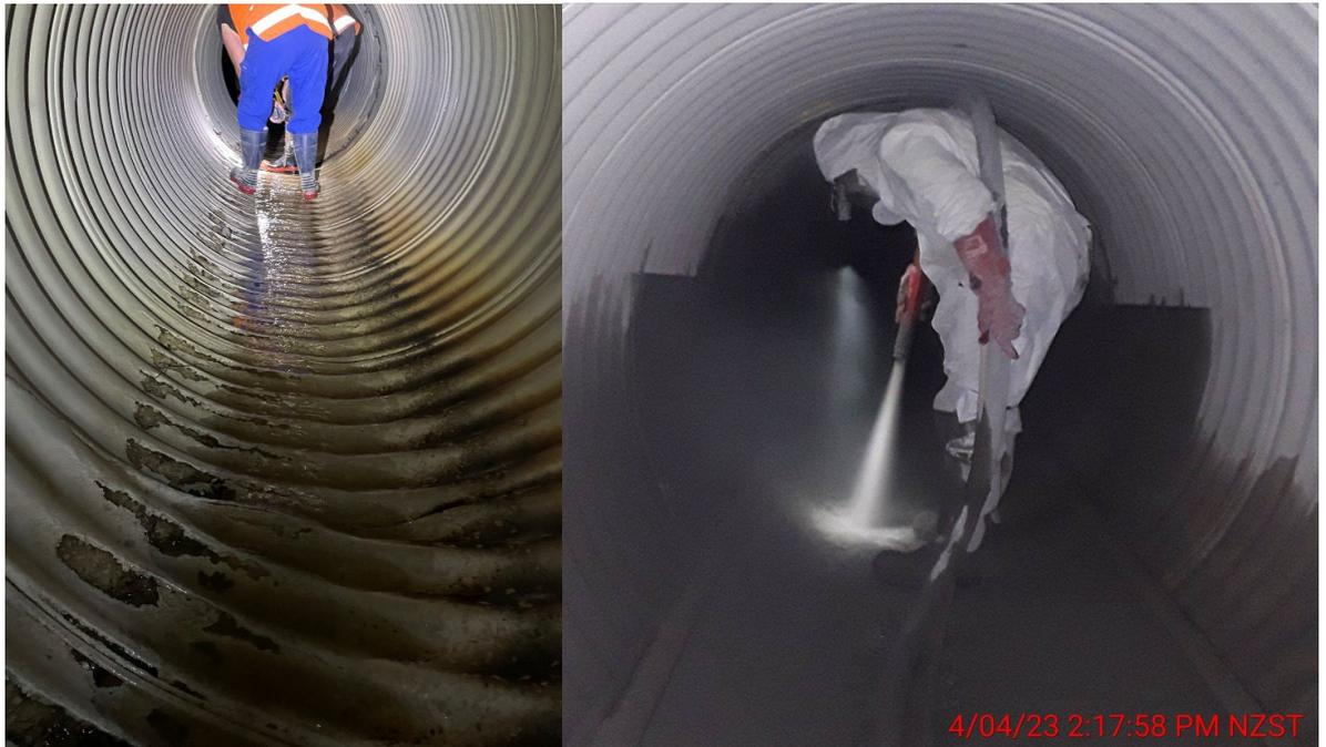
*Site 17 Seton Nossiter culvert repair, showing damaged culvert and repair work in progress*
