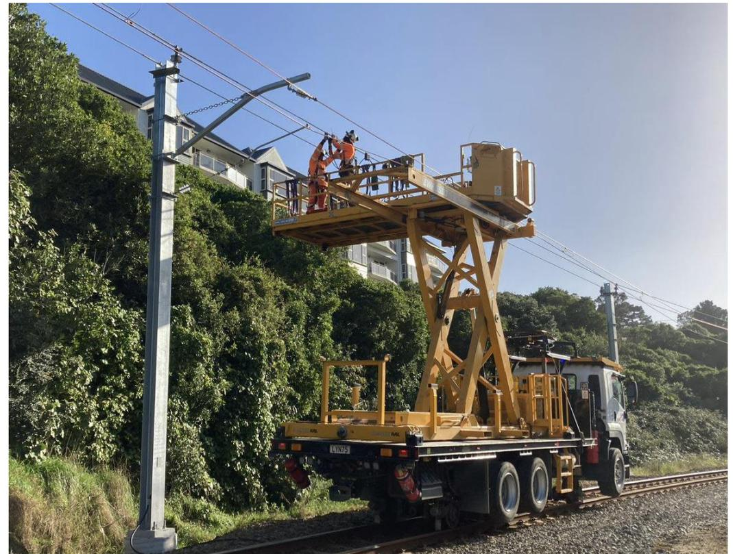
*Easter Block of Line Activity- Raroa Station pedestrian bridge and ongoing removal of redundant traction masts and defect remediation*
