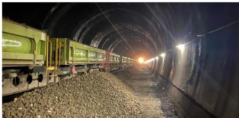
*New bottom ballast layer dumped ready for excavators to initially spread, and Posi-Track and surveyors to bring to design level*
