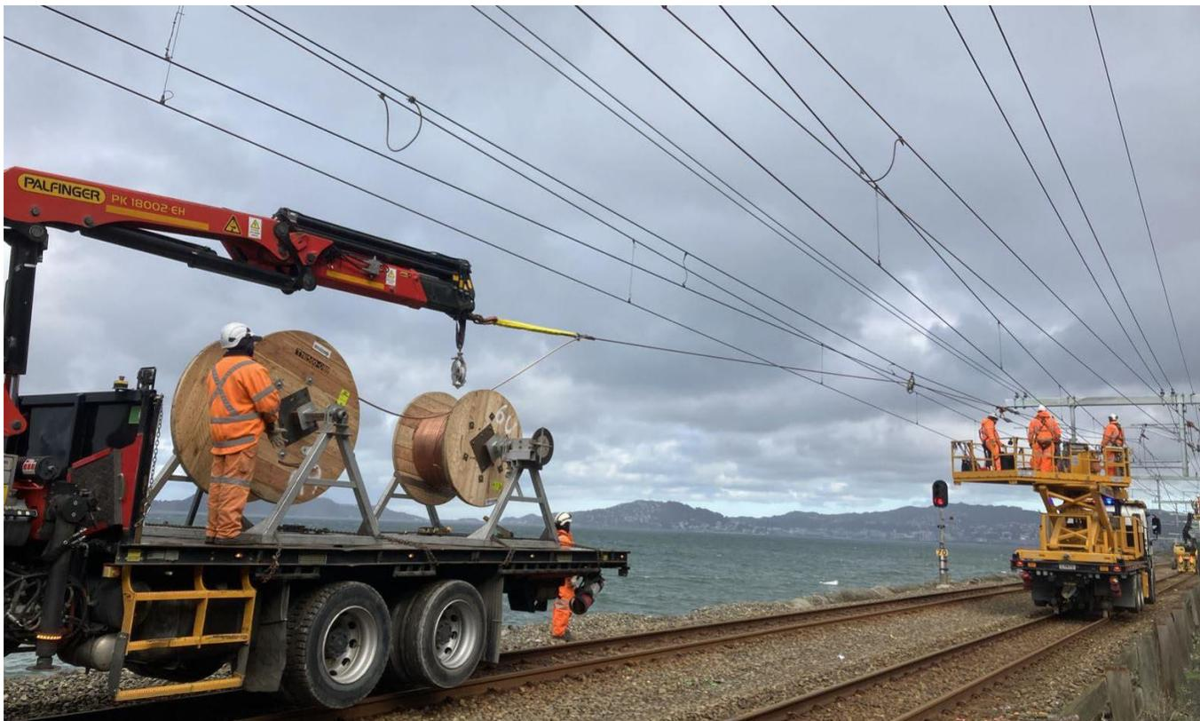
*New (Catenary and Contact) wire installation on the UP Main replacing the existing old ones*
