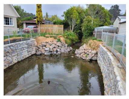
Figure 7 Redi-Rock walls and scour protection upstream of Sunbrae Culvert (photo credit: GHD)
