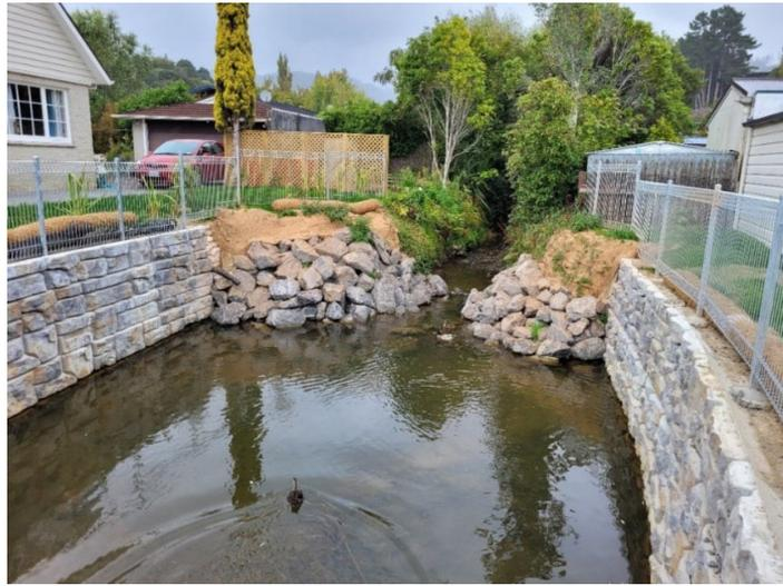
**Figure 9 Redi-Rock walls and scour protection upstream of Sunbrae Culvert (photo credit: GHD)**
