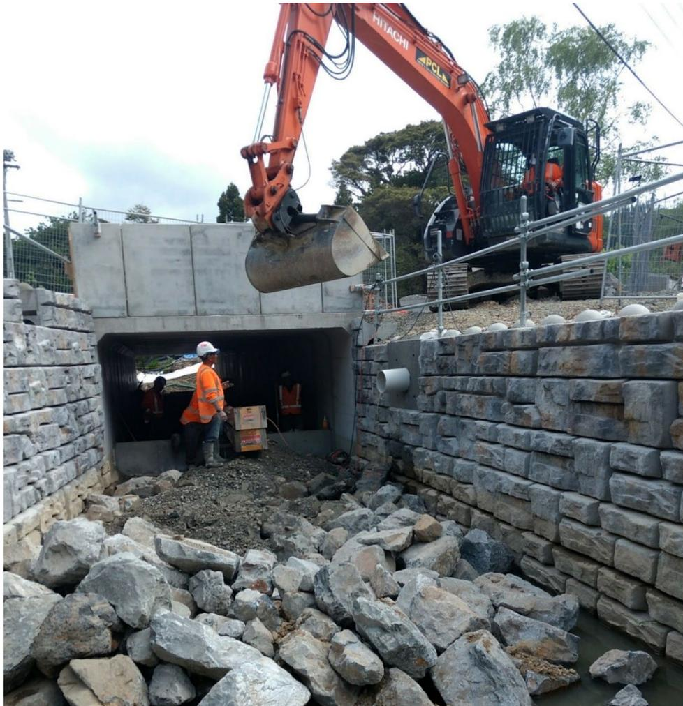
**Figure 10 Placement of stream bed material within Pinehaven Culvert using conveyors (photo credit: GHD)**
