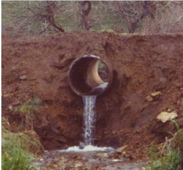
**Figure 19: Perched culverts like this do not allow passage of fish.**
