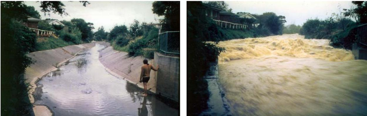
**Figure 3:** Channel lining and high flood flows in 1975 in Wairau Creek (North Shore, Auckland).
