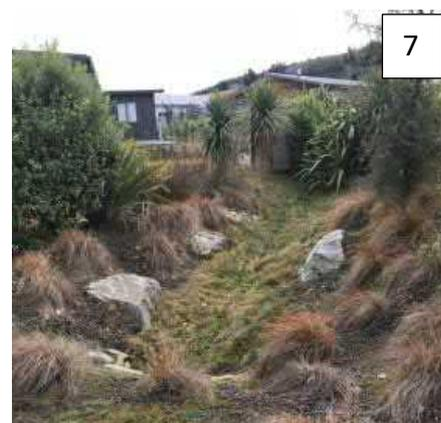
**Photo 5:** Raingarden with unplanted stone mulch and exposed overflow dome.
