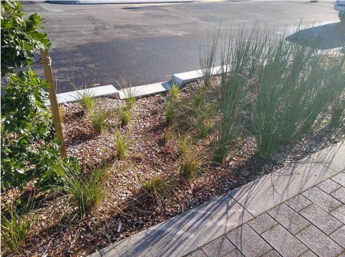
**Figure 15. Raingarden treating road runoff.**
