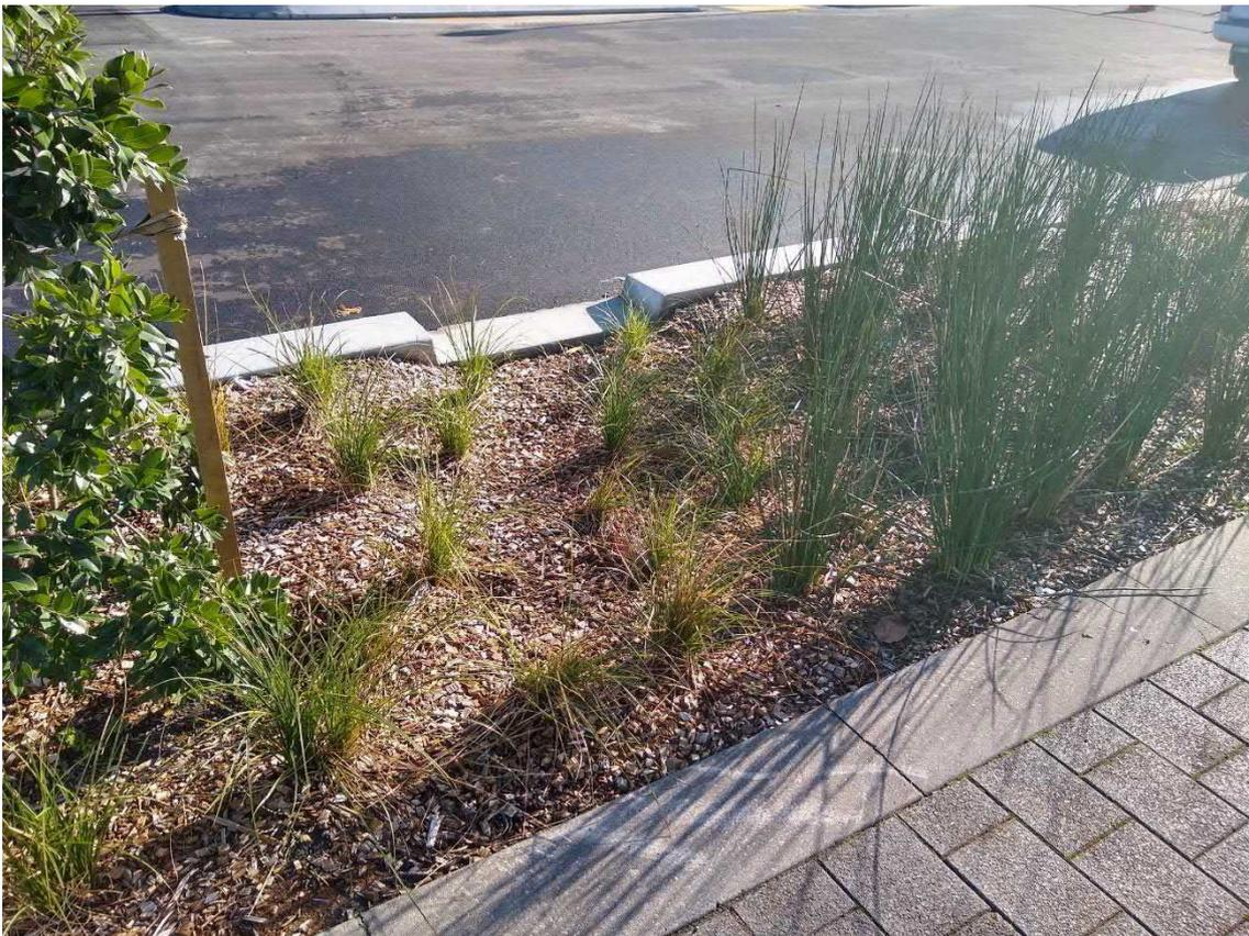
**Figure 15. Raingarden treating road runoff.**
