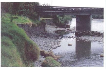
PHOTOGRAPH 7: FURTHER UNDERMINING OF THE STATE HIGHWAY 1 BRIDGE PIER, April 1998
