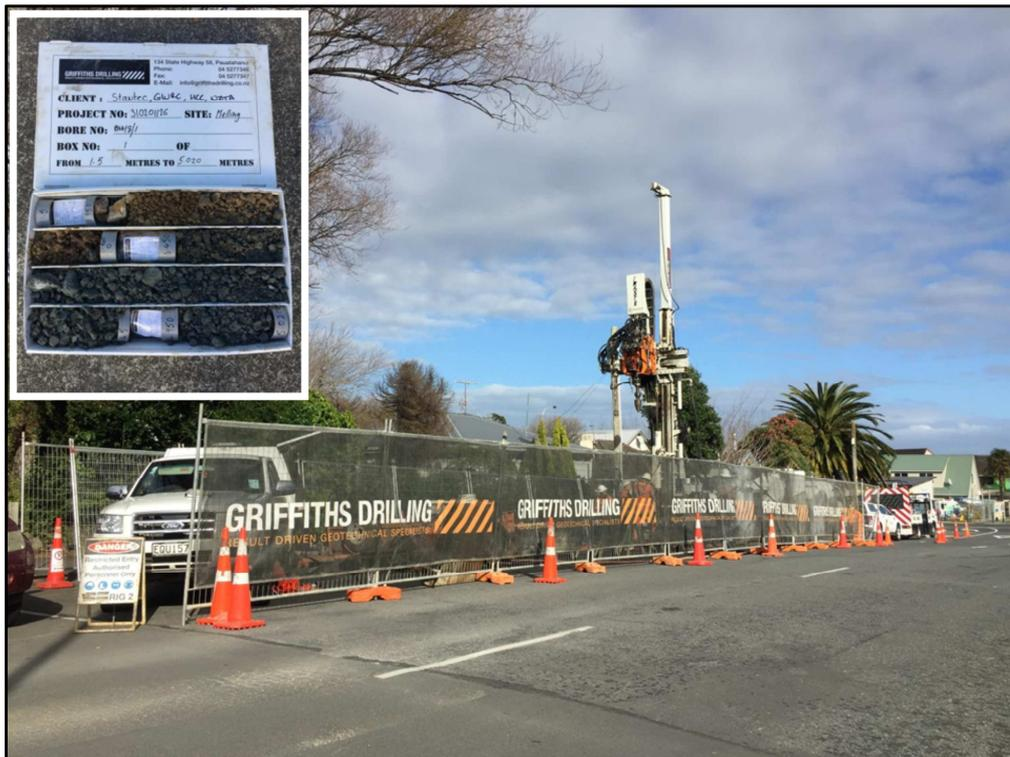
Work to assist with design and future consents for the RiverLink construction. We are looking for the aquifer, Wellington Fault Line and below ground material types. Where the aquifer is found we will be installing monitoring equipment to provide information about the changes in pressure within the aquifer and ground above it.
