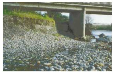
Photograph 6: Undermining of the State Highway 1 bridge pier, left bank, June 1997
