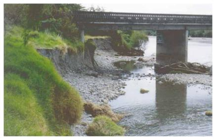
Photograph 7: Further undermining of the State Highway 1 bridge pier, April 1998
