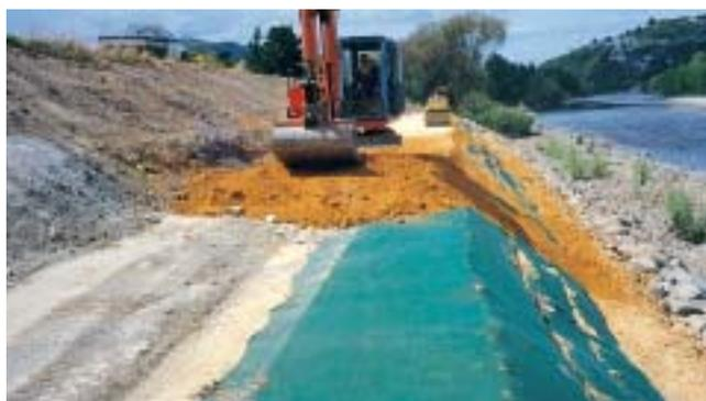
Repairing a stopbank and constructing new bank-edge protection at Manor Park, Lower Hutt.
