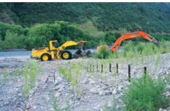
Willow plantings reinforced with rail-iron debris fences, being used to reinstate eroded river bank and berm areas at Manor Park, Lower Hutt.
