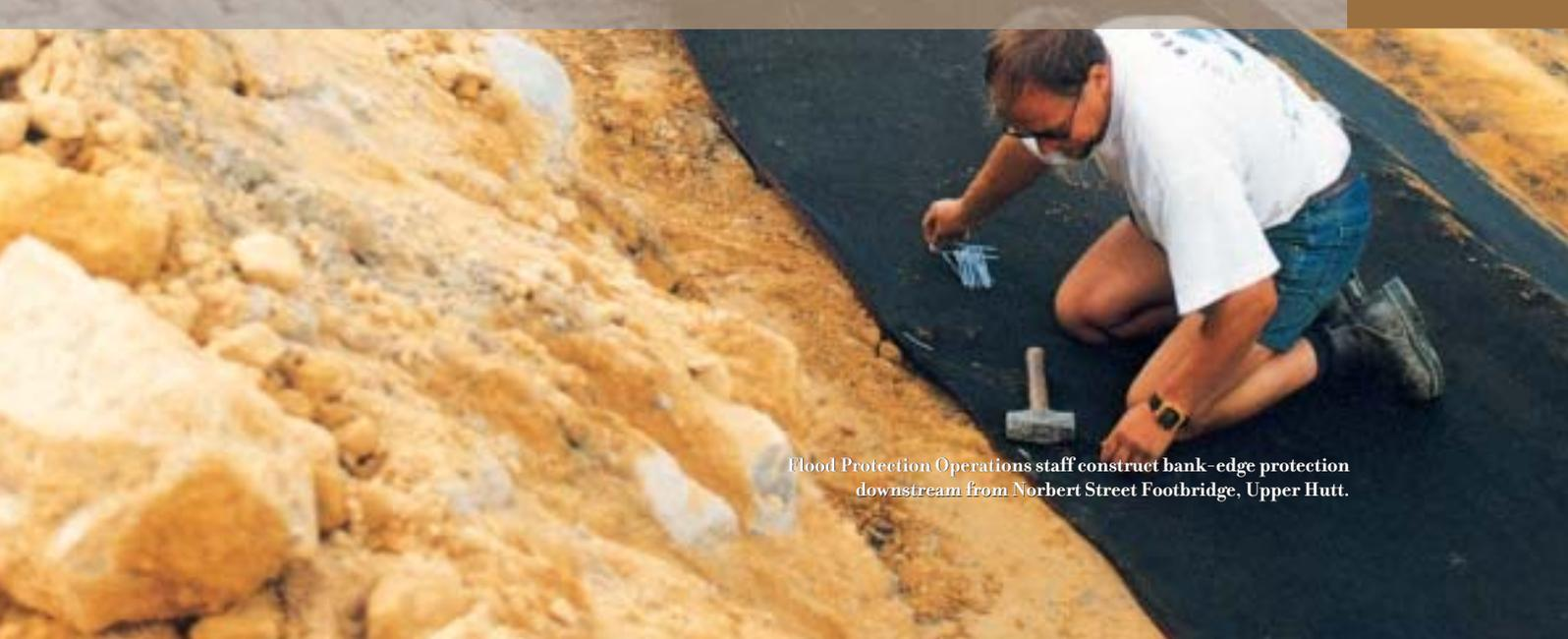
Flood Protection Operations staff construct bank-edge protection downstream from Norbert Street Footbridge, Upper Hutt.
