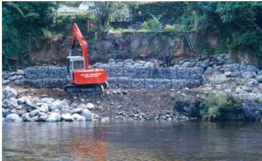
A digger works to place gabion baskets and rocks against an eroding bank at Bridge Road, Upper Hutt. Residential homes sit just beyond the eroded river edge.
