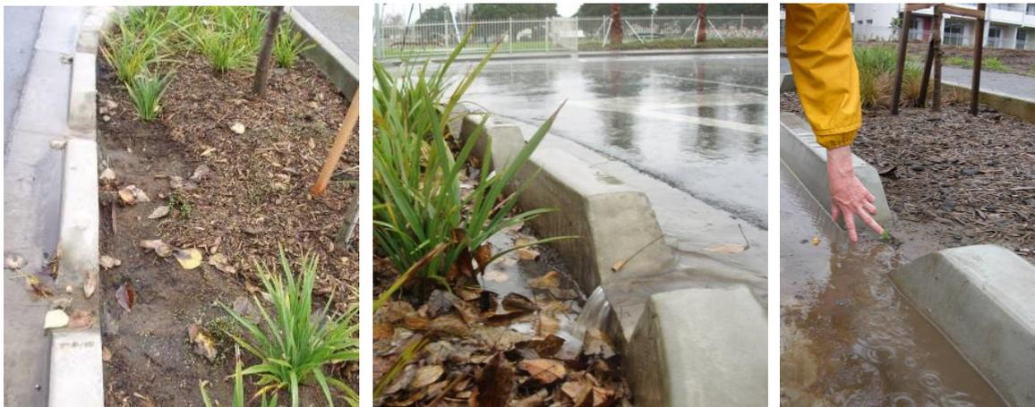
Scouring at raingarden inlets displaced mulch and soil (left). Stormwater inflow showing concentration of water to one side of the cut, but no scouring or leaf litter displacement (centre) and stormwater prevented from entering the raingarden due to overfilling with media/mulch (right). All photos in June/July 2008.
