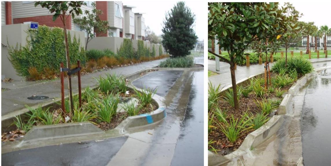
The combination of inlet placement and gutter design means most runoff bypassed this rain garden, so overloaded the next raingarden; blue marks indicate where new kerb cuts were to be made (left) 2008. Newly renovated raingarden with c. 150 mm of media removed except around retained trees and plantings, e.g. dense flax at the far end. New inlets improve flow from the street gutter (right) 2008.
