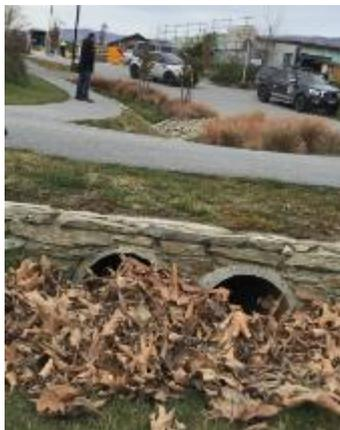
The most frequent maintenance activity is mowing grassed swales and removal of any debris in the swale systems (including slotted weir controls, pipes and cesspit inlets), approximately two-monthly, followed by trimming of hedges (although most hedges in the road reserve are maintained by adjacent owners); mowing frequency is likely increased where adjacent owners use irrigation (and fertiliser). At least annually (or after significant rain events) the following occurs:
