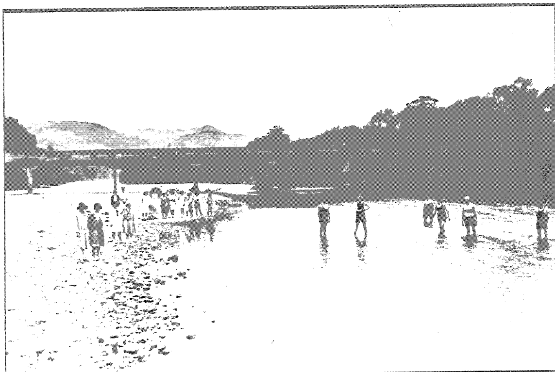
Plate 82: Moonshine Bed Levels, 1931. Source: Alexander Turnbull Library neg. G46227
