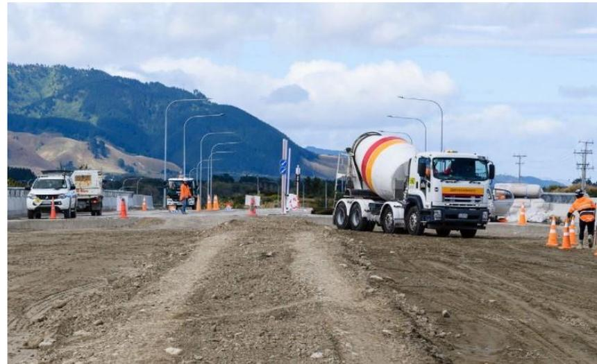
Working on the subgrade (bottom) layer of the new road
