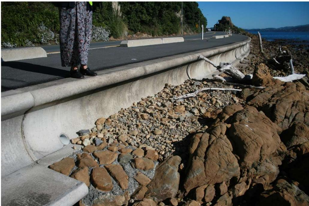
**Figure 3** *Unnatural transition from sea wall to rocky beach (to be avoided). The squared off end of the tread dominates the rock. It would have improved this transition if a large rock or a few large rocks were partially cast in to the end of the tread with minimal visible grouting (as opposed to here where the rocks set in the concrete matrix appears highly unnatural). Photograph by J. Head May 2, 2019.*
