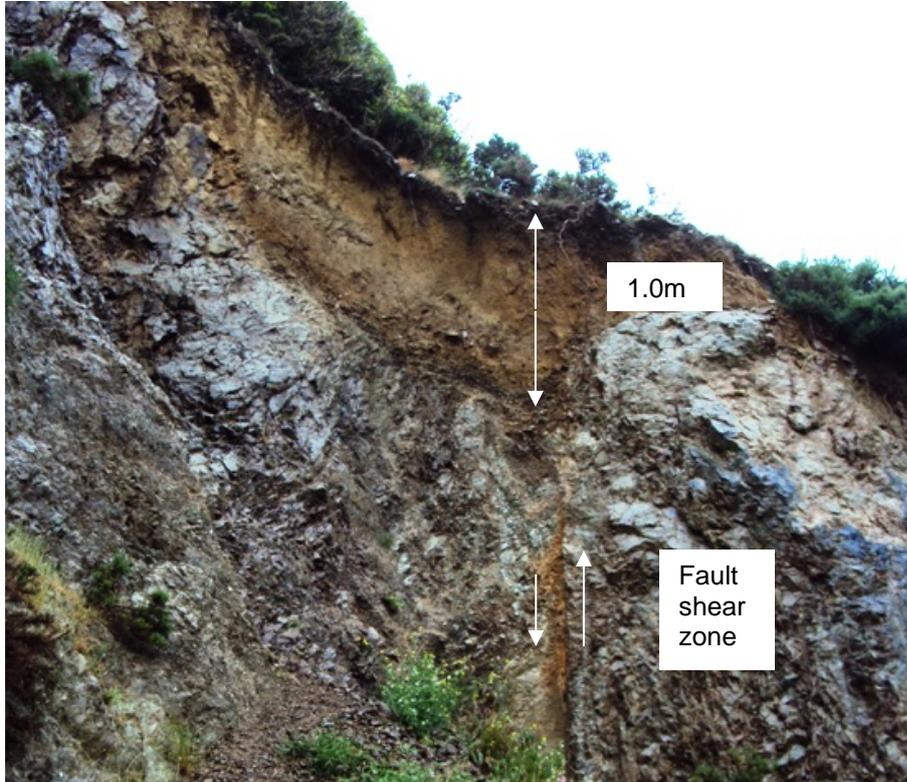
Plate 3-5 Fault shear zone on eastern access road cut slope
