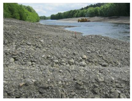
Figure 10: 'Wet' gravel extraction: bulldozer forming low flow channel
