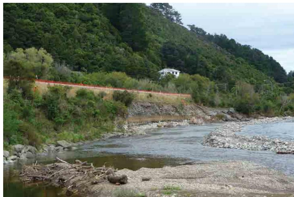
*The river has eroded the bank adjacent to SH2, affecting the Hutt River Trail. Erosion protection work by NZ Transport Agency has been carried out to prevent further undermining.*
