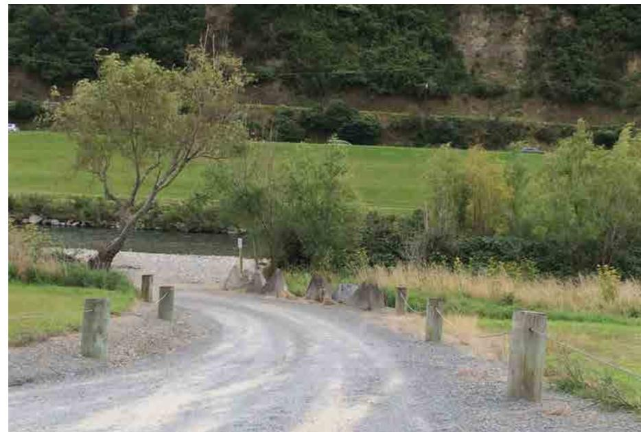
Vehicle access to Taita Rock swimming hole, with bollards and wire rope barrier to prevent vehicles driving on the river berm
