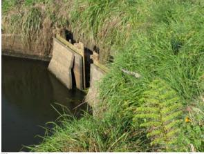
**Figure 3d.** Looking upstream at the old-style flap valves that protect the southern tributary.
