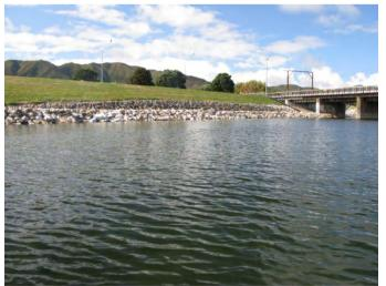
**Figure 17.** Looking downstream at a section of the Hutt River that is protected by anit-scour
