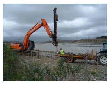
Debris fence construction (driving irons) – Ōtaki River
