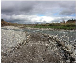
Temporary vehicle access track on river bed, formed by blading with a bulldozer
