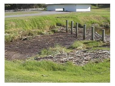
Debris arrester (timber poles) across Waimeha Stream
