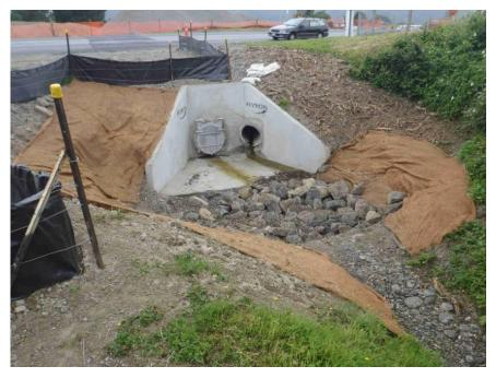
Silt fencing and ground stabilisation around newly installed wingwall
