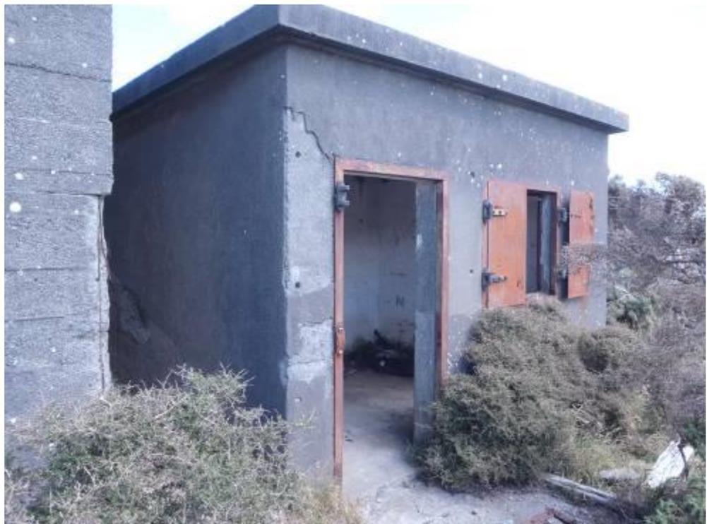
Figure 30: The wireless room. The reinforced concrete walls were rendered on the outside. The shutters are still in place and at the bottom of this photograph there is visible a small portion of the door which currently rests on the ground in front of the building.
