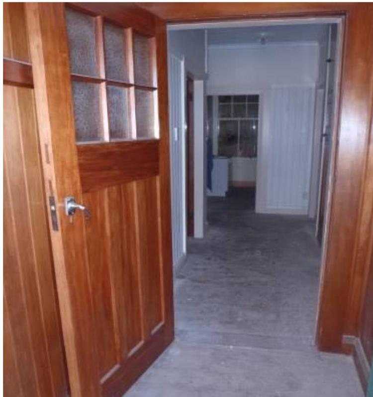
Figure 16: Interior of Number One Lighthouse Keepers' House showing vestibule, hall and tongue and groove wood panelling.
