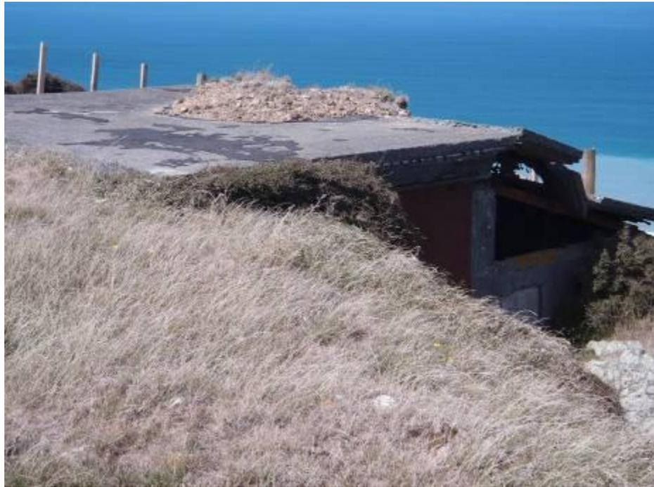
Figure 27: The observation post, built of reinforced concrete. Inside is the concrete foundation of what might have been a range finder or telescope. This building retains part of its camouflage (a layer of earth and vegetation visible on its roof) but the cantilevered roof over the viewing slit has collapsed. The path that has been constructed to allow entry to the building is shown to the right of the photograph
