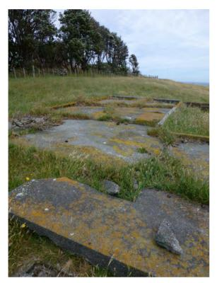
Lichen and mold on concrete foundation
