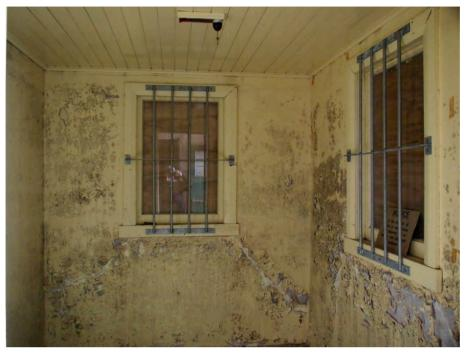
South west corner room, peeling paint and cracked plaster
