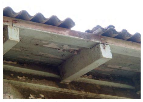
Damaged asbestos roofing - west elevation
