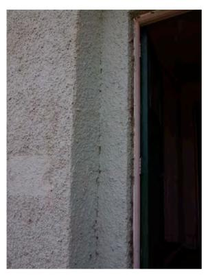
Cracking to corner, west elevation
