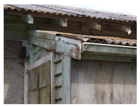
Paint peeling, cracked asbestos roofing, algae growth - typical of all elevations
