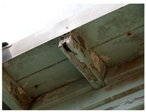
Rotten rafter end, rusting nails, peeling paintwork – west elevation
