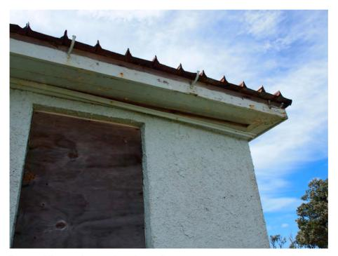
Loose molding, rusting trough section roofing
