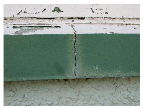
**Cracked sill, west elevation**
