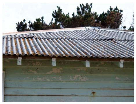
Lifting asbestos roofing – east elevation
