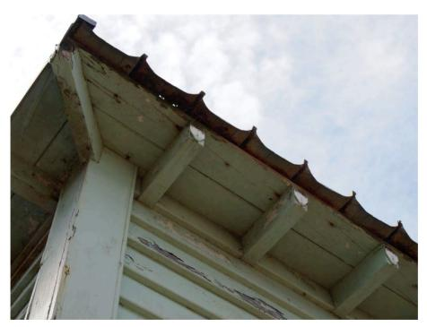
Rusting underside of the trough section roofing – south west corner
