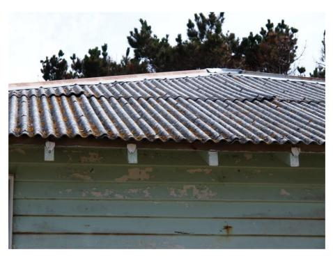
Lifting asbestos roofing – east elevation
