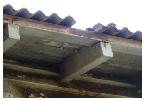
Damaged asbestos roofing - west elevation
