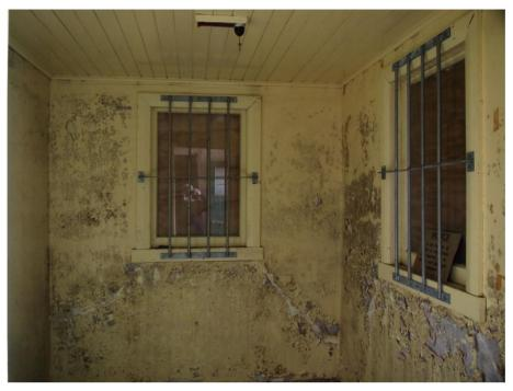
South west corner room, peeling paint and cracked plaster
