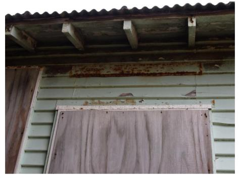
Rusting head flashings, peeling paint, missing guttering – typical of all elevations
