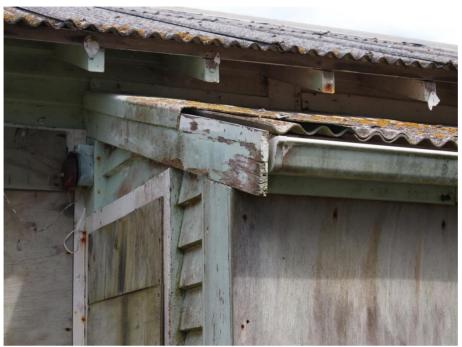
Paint peeling, cracked asbestos roofing, algae growth - typical of all elevations
