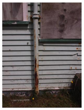
Rusting vent pipe, rusting nails and split and damaged weatherboards – east elevation
