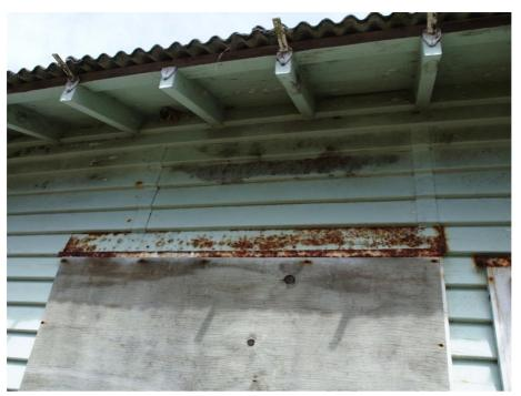
Rusting head flashings, missing guttering, fraying corrugated as bestos roofing edging – east elevation  $\,$
