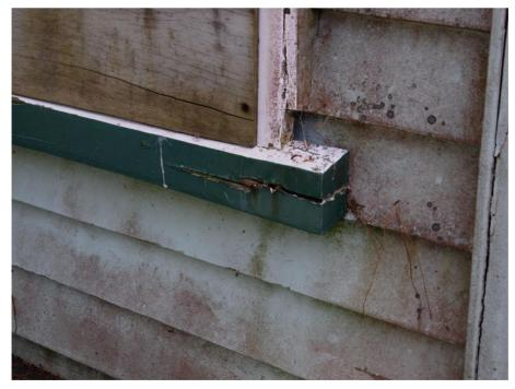
**East elevation splitting sill**
