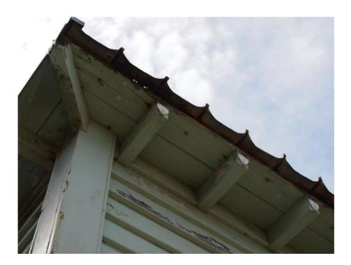
Rusting underside of the trough section roofing – south west corner
