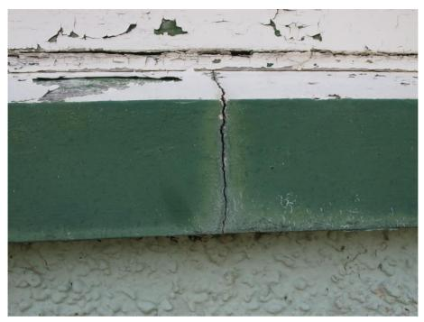
**Cracked sill, west elevation**
