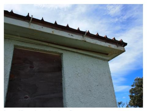
Loose molding, rusting trough section roofing
