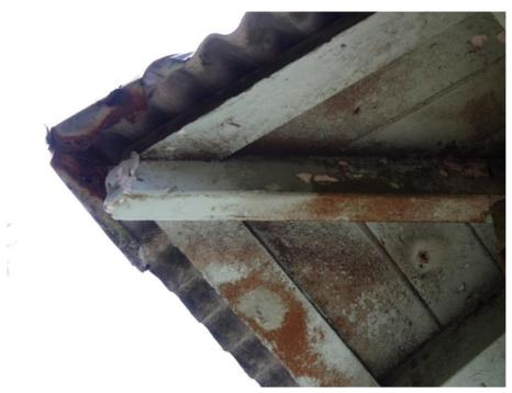
Rusting under side of corrugated steel ridge flashing – west elevation
