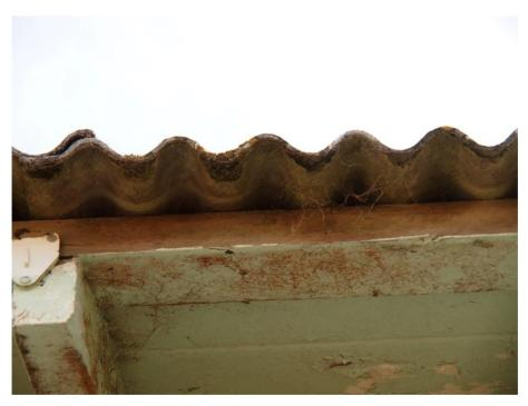
Fraying cut edges to roofing – east elevation
