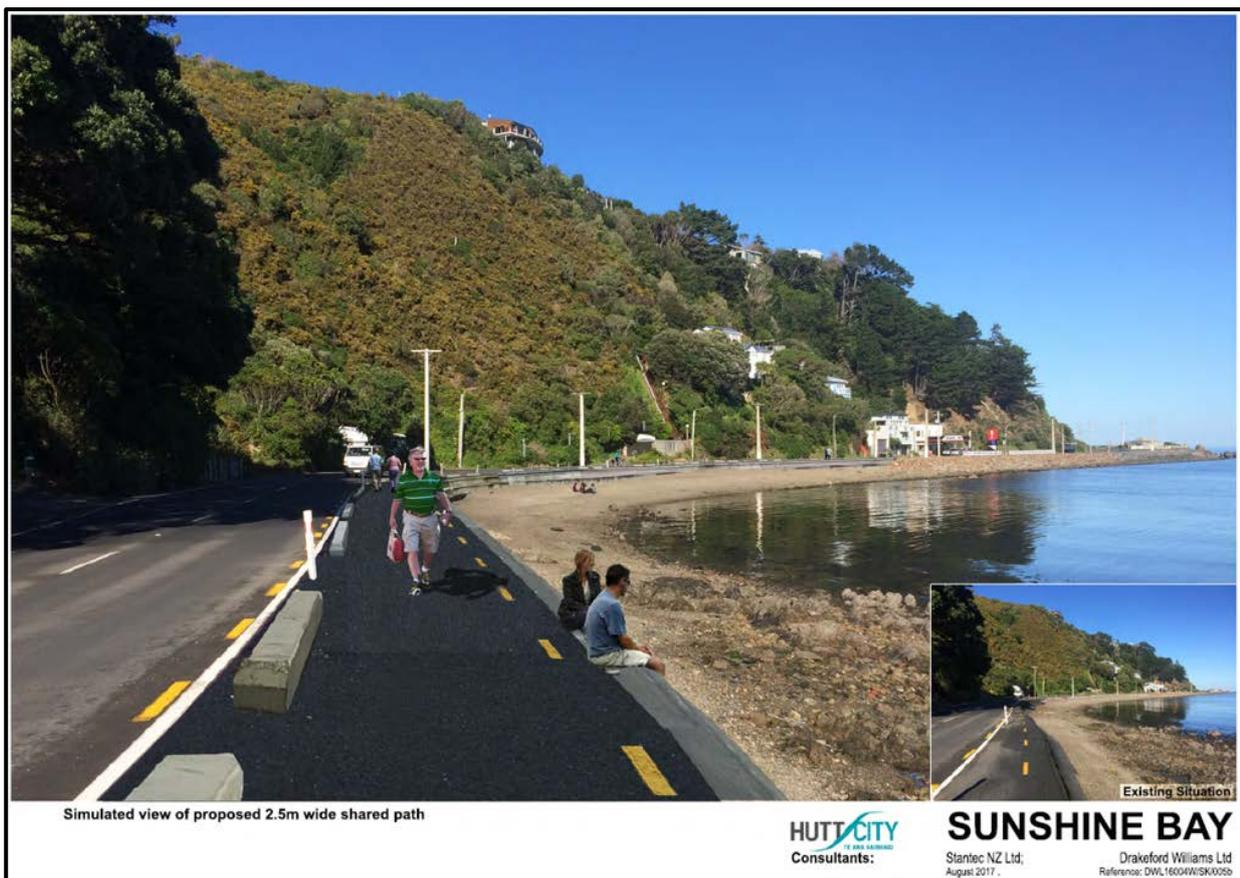
Figure 1-1: Proposed shared path showing a typical widening
