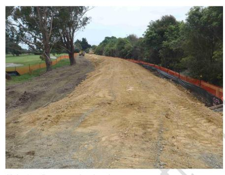
Silt fencing adjacent to earthworks on berm
