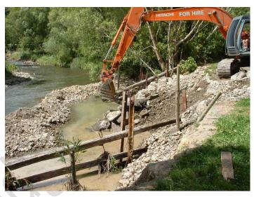
Repairs to timber permeable groynes on the Wainuiomata River. Note the separation of the work area from the wet channel through the use of bunding
