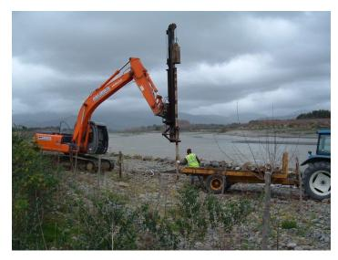
Debris fence construction (driving irons) – Otaki River
