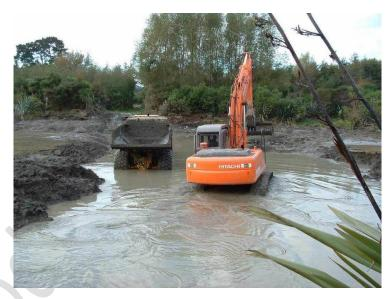
Silt excavation in Chrystalls Lagoon. Note use of self-draining weed bucket
