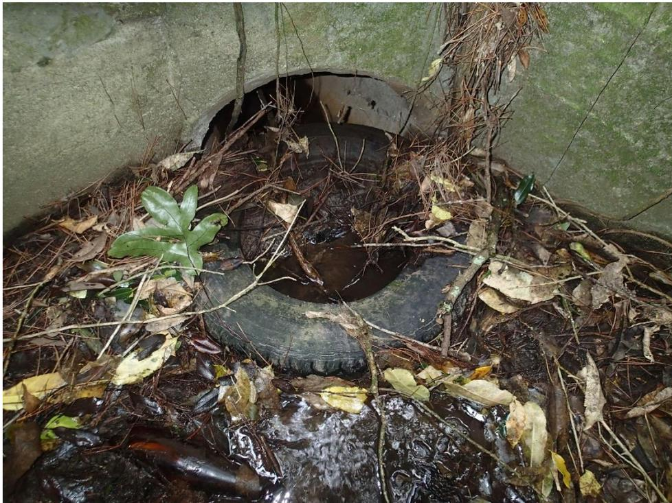
**Figure 1. Culvert inlet (partially blocked) with wingwalls**
