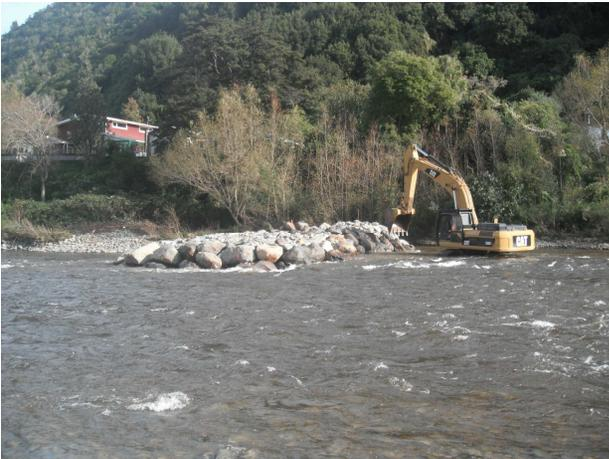
*Groyne placement. Machinery working close to bank edge to minimise disturbance to the riverbed*
