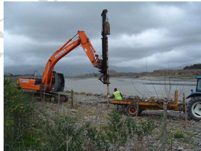
*Debris fence construction (driving irons) – Otaki River*
