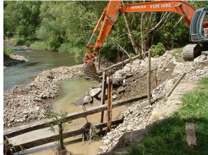
*Repairs to timber permeable groynes on the Wainuiomata River. Note the separation of the work area from the active channel through the use of bunding*
