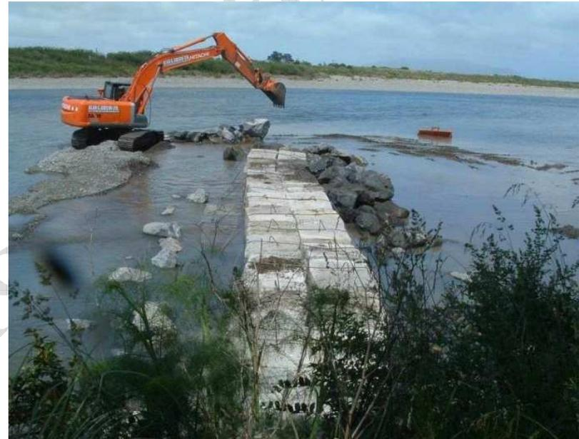
*Groyne construction, showing use of bunding to protect works from flowing water and use of a formed working platform to elevate machinery out of flowing water*
