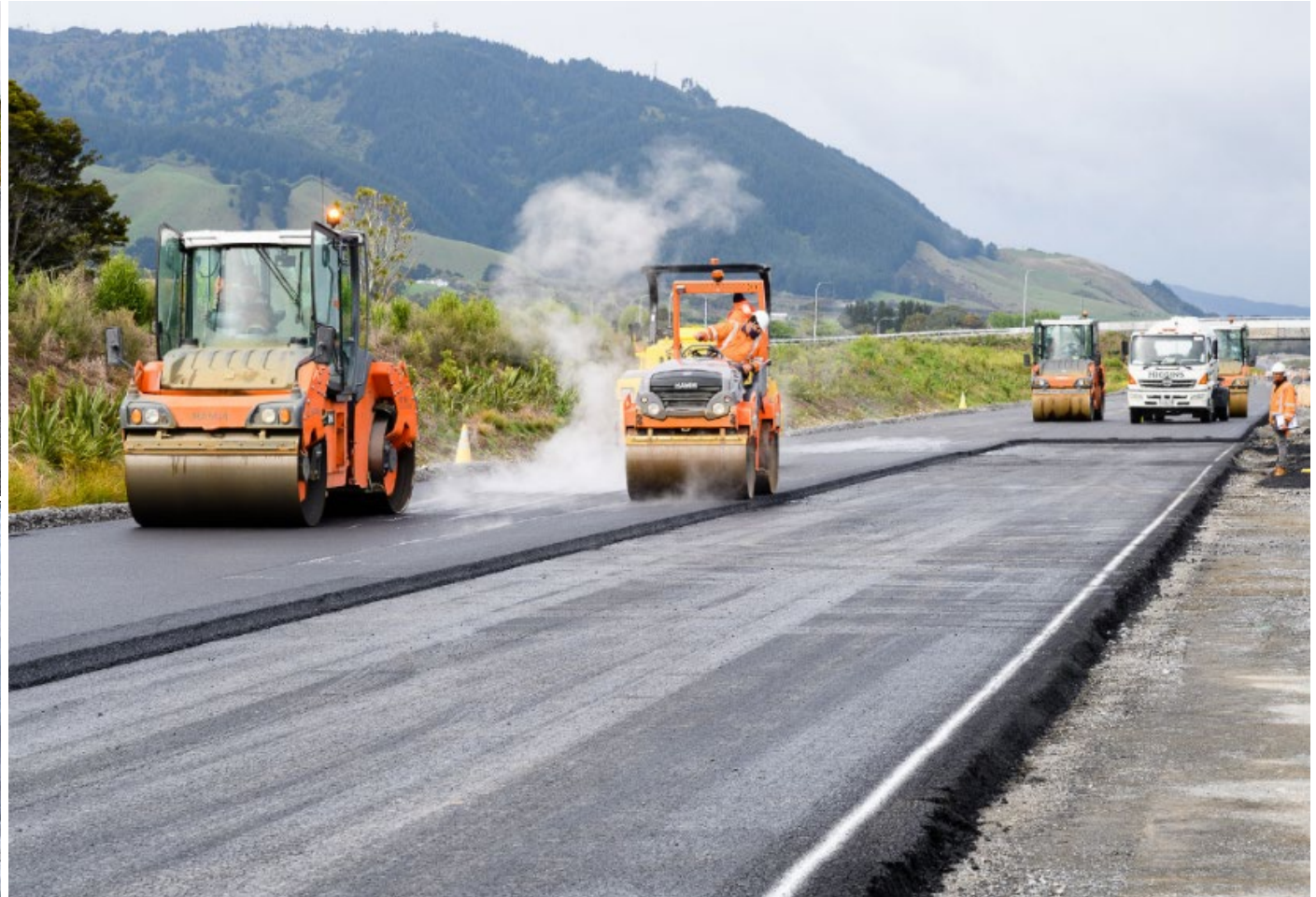
Pavement works on southbound lanes, near Te Horo
