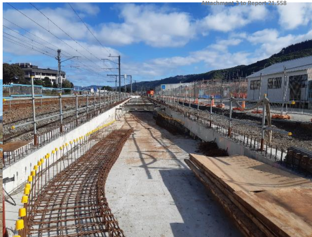
Ramp at Petone underpass taking shape
