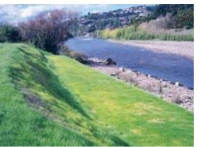
The finished product. Grass takes hold on the repaired stopbank and berm at Manor Park.
