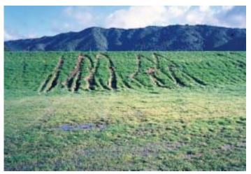
Careless use of vehicles has resulted in deep tyre ruts on the stopbank at Totara Park, Upper Hutt. Damage like this can seriously affect the flood defences' performance during a flood.
