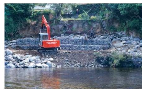
A digger works to place gabion baskets and rocks against an eroding bank at Bridge Road, Upper Hutt. Residential homes sit just beyond the eroded river edge.
