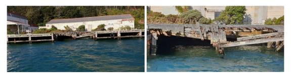
Photograph One and Two: Pictures of collapsed Shelly Bay wharves.
