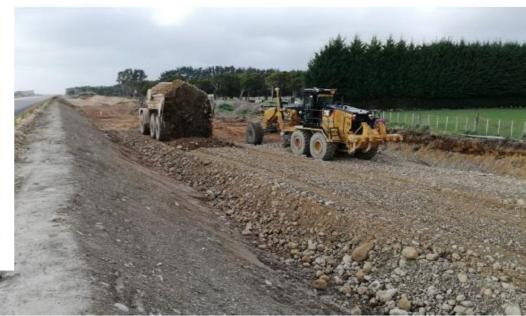
Picture 2 - Placement of gravels for the subgrade of Winiata Link Road.
