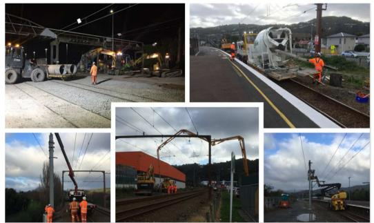
KiwiRail project teams work on excavating pole foundations, pouring concrete in various locations and erecting new traction masts.
