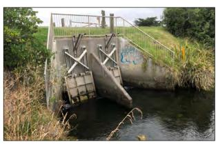
Flow control gates on the streams entering the northern lagoon
