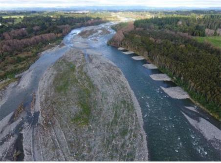
Waingawa River gravel groynes constructed to protect against erosion into the buffer area of native trees.
