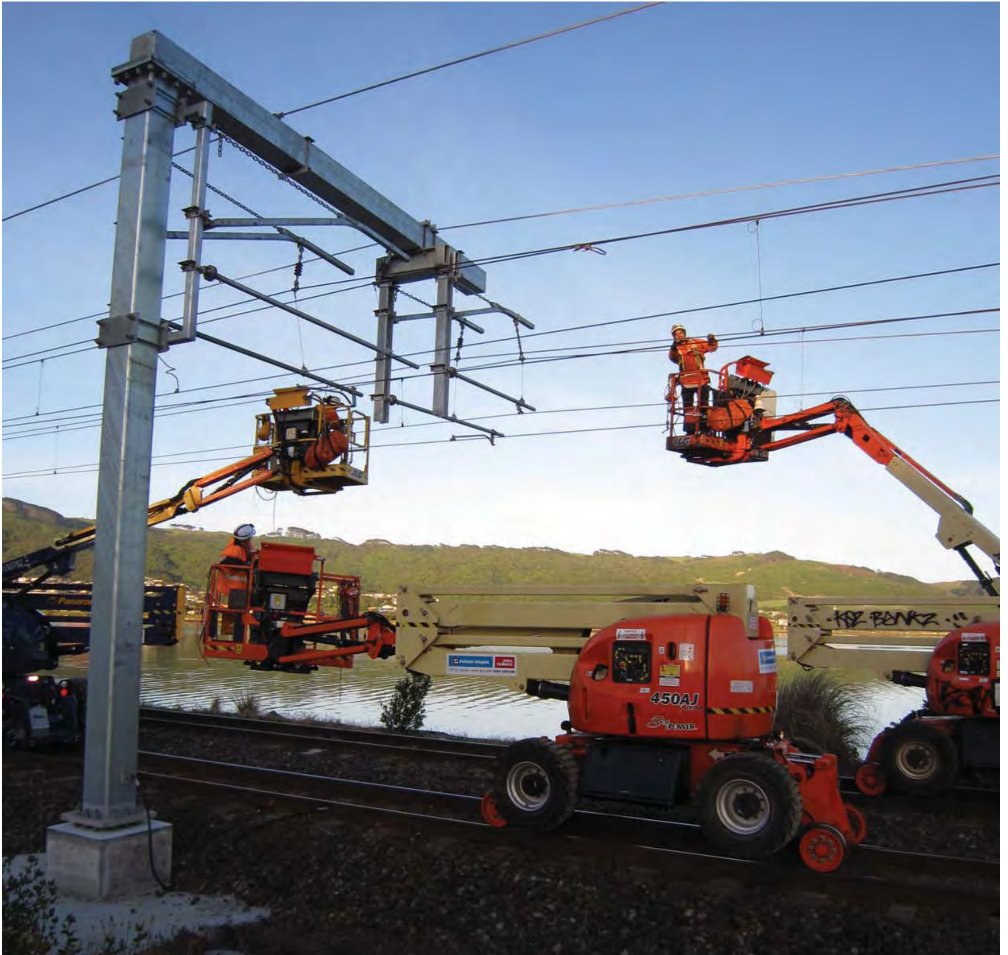
Works at Porirua replacing overhead traction cables
