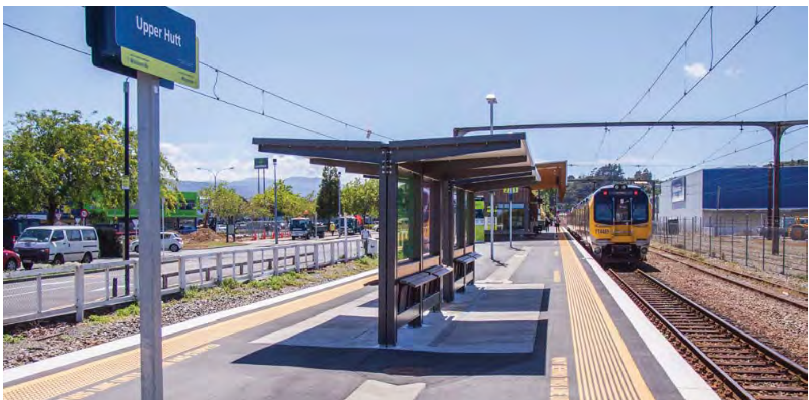
New Shelter at Upper Hutt Station
