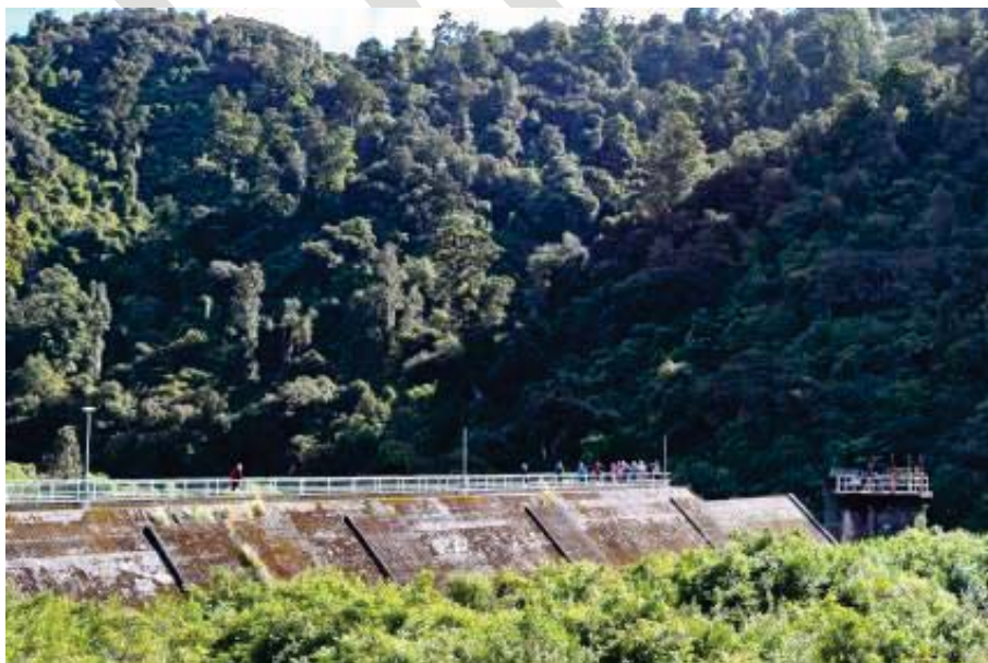
Caption: Guided walking tour viewing Moreton Dam. Construction of this dam was completed in 1911 and it was decommissioned and superseded by the Te Marua lakes scheme in 1988. The dam is historically significant because of its form of construction which is unusual in New Zealand; reinforced concrete made in sections of slab and buttresses.
