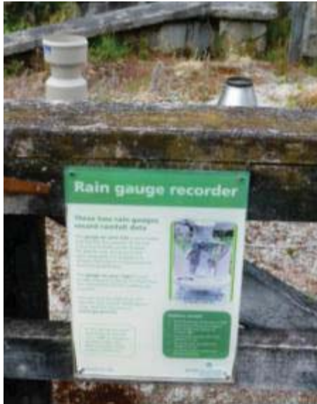
Caption: Telemetered rainfall gauge near Morton Dam, Wainuiomata (photo FC)
