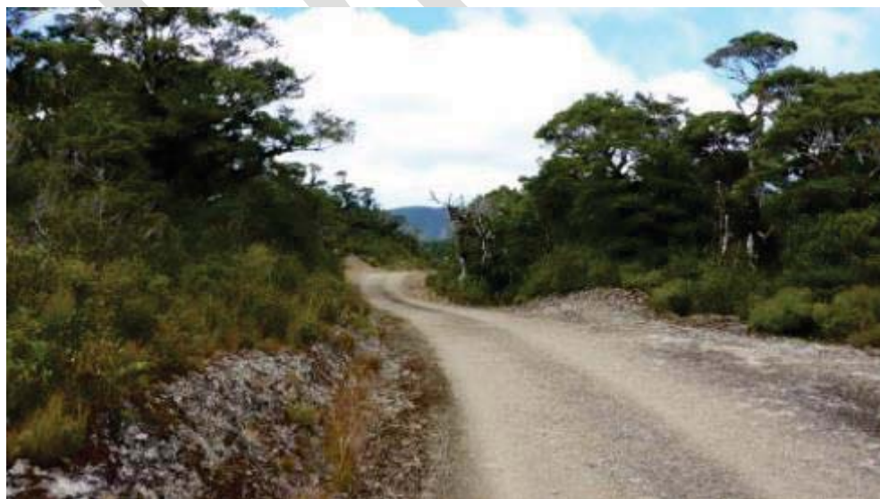
Photo: Orongorongo road is a key asset providing management access into the remote Orongorongo water catchment. Following a ridge line, it is frequently snow covered in winter (Photo FC)
