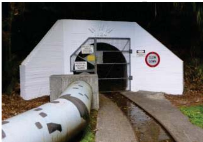
Caption: The three kilometre long Orongorongo Tunnel provides access for water pipeline inspections and maintenance. It runs from the Big Huia Creek Intake in the Orongorongo Catchment through to the George Creek area of the Wainuiomata catchment. A diesel engine and cart carry gear and equipment. Glow worms live in the tunnel and can be seen approximately 30m from the tunnel entrance. (Image: FC & GWRC collection)
