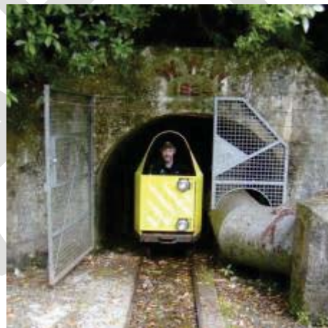
Caption: The three kilometre long Orongorongo Tunnel provides access for water pipeline inspections and maintenance. It runs from the Big Huia Creek Intake in the Orongorongo Catchment through to the George Creek area of the Wainuiomata catchment. A diesel engine and cart carry gear and equipment. Glow worms live in the tunnel and can be seen approximately 30m from the tunnel entrance. (Image: FC & GWRC collection)
