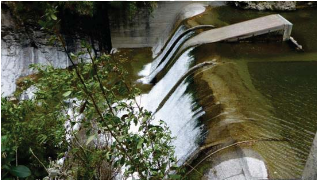
Caption: Kaitoke Water Works Weir location of the water intake on the Hutt River constructed between 1946 and 1957 and refurbished on a number of occasions since then. There are two tunnels associated with the weir. (Image FC)
