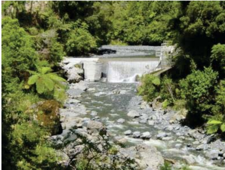
Caption: Orongorongo Weir and water intake, Orongorongo River. Assets such as weirs are being progressively seismically strengthened via asset renewal programmes.
