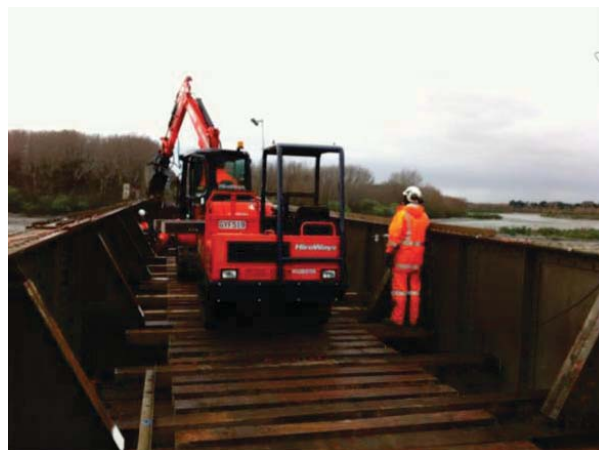
Bridge 52, Waiohine River
