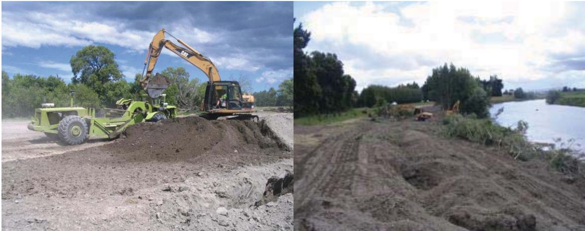
Ruamahanga River berm lowering adjacent to Martinborough ponds
