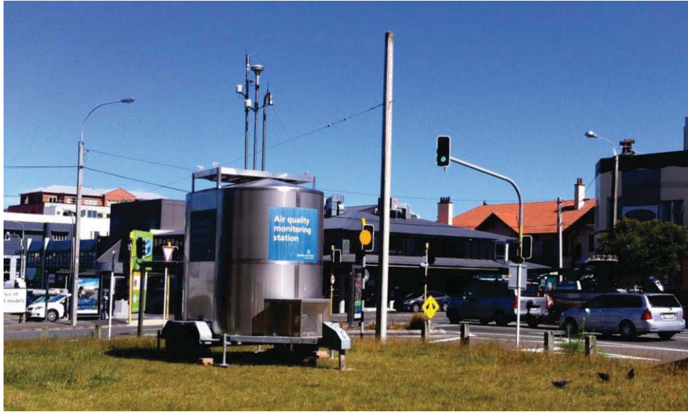
Mobile monitoring station on the new site at the corner of Willis Street and SH1
