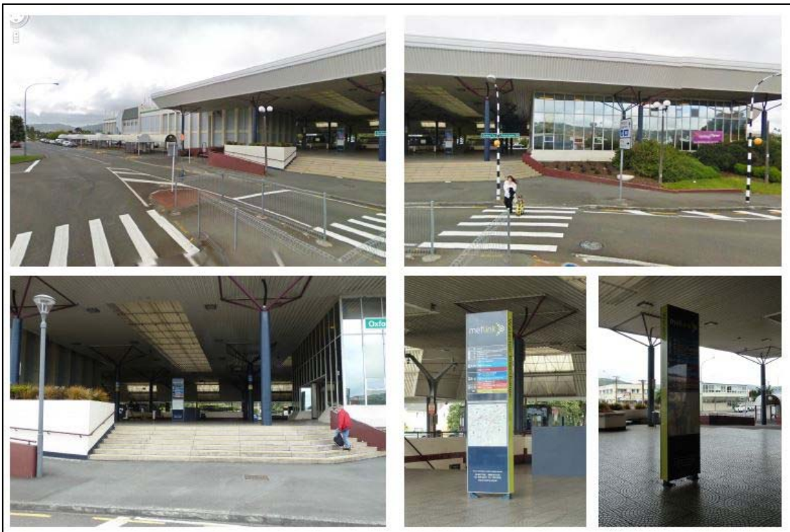
Image 3: Lack of external signage at Waterloo Station
