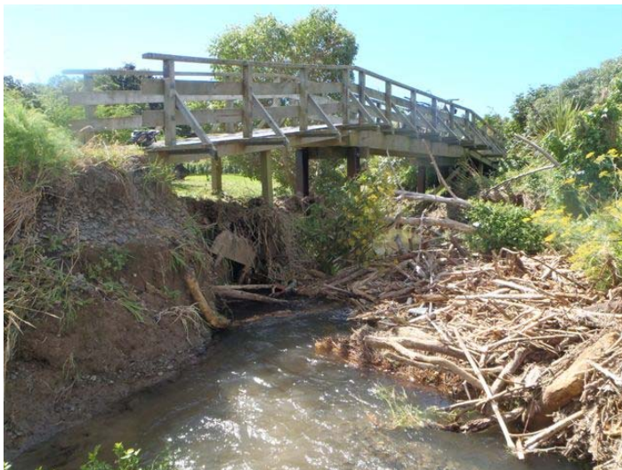
Bridge over Wainui Stream, Queen Elizabeth Park
