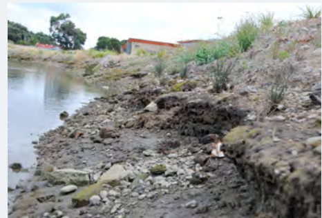
Bank erosion in the lower Waiwhetu Estuary showing the loss of remediation capping and plantings.
