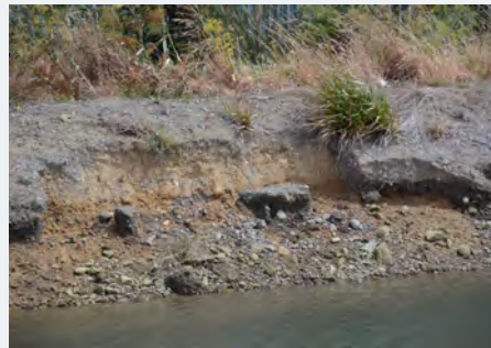
Bank erosion in the lower Waiwhetu Estuary showing the loss of remediation capping and plantings.
