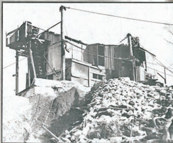
Bagnuda, Adams and Blyth crusher erected upstream of Ewen Bridge 1930, photo 1958 Alexander Turnbull Library
